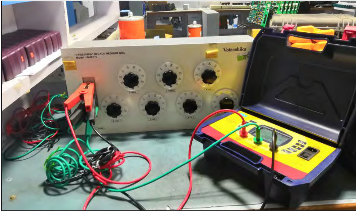
Calibration setup of a Decade Megohm Box for Insulation Tester Calibration
